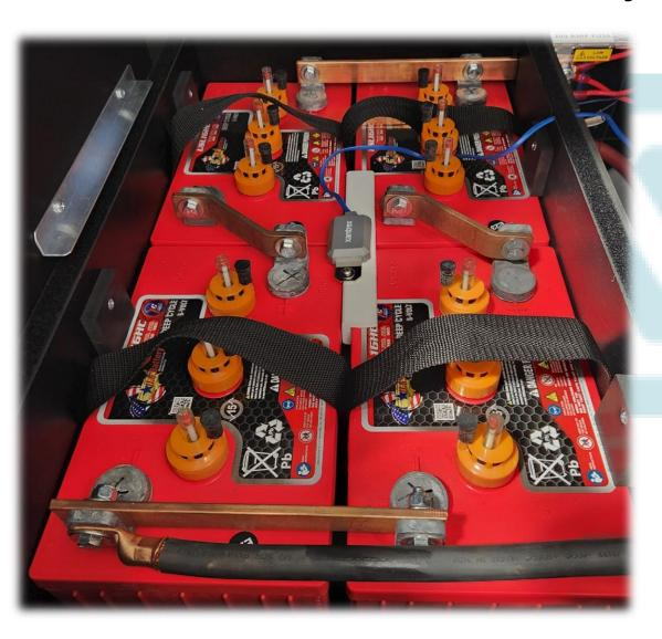
Check the water level of each battery monthly. If, you are having to add more than one gallon of water every month, you should start checking/adding water weekly and expect to replace your batteries soon.
